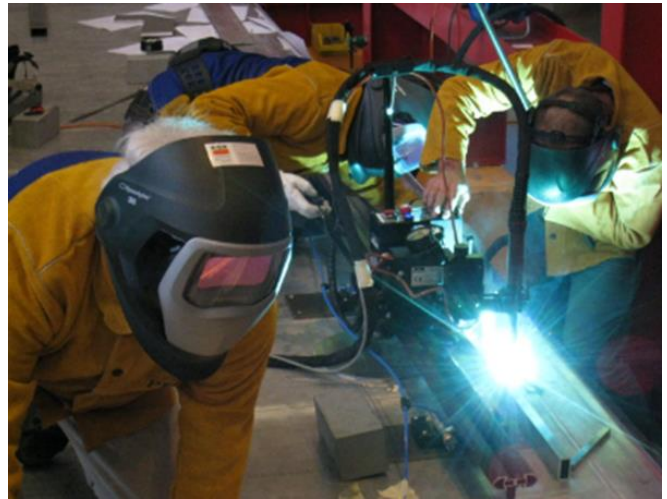
Fig. 6. First pass weld of one of the panels.
