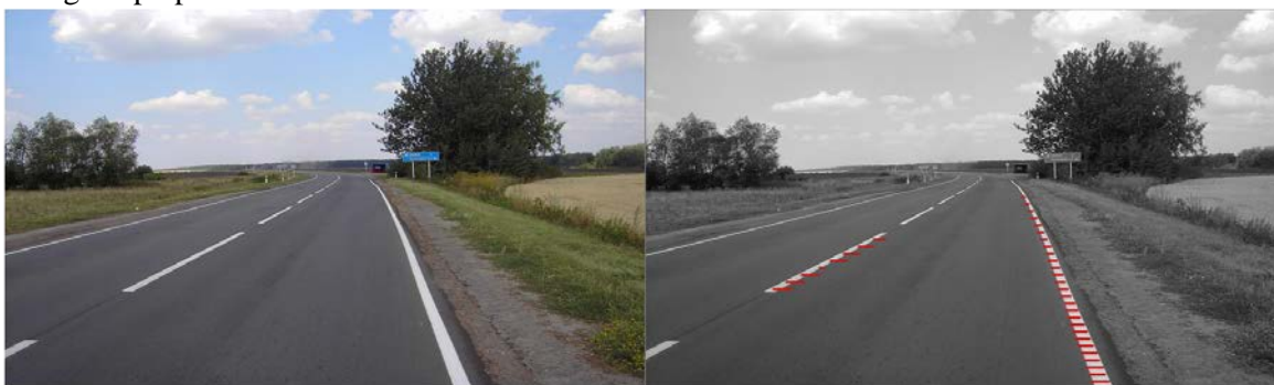
Figure 6. An example of finding a road marking.
