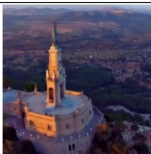
Figure 8. Image after restoration.
