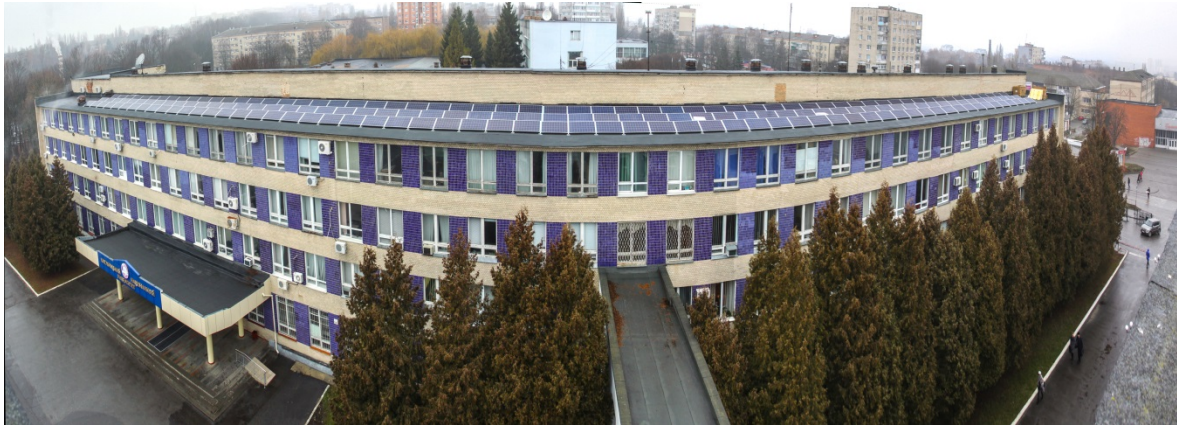
Figure 5: Rooftop solar power station of Khmelnytskyi National University
