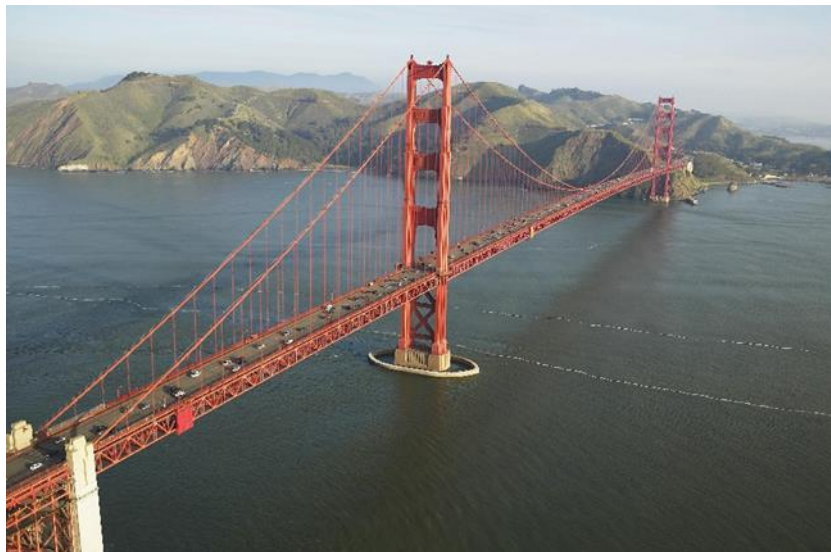
Figure 1: The example of replacing bending with stretching and clamping is suspension bridge
